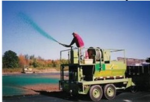
APPLYING HYDROSEED
